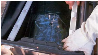
**2d** Install cut pipes x 2 into holes in top of box.
